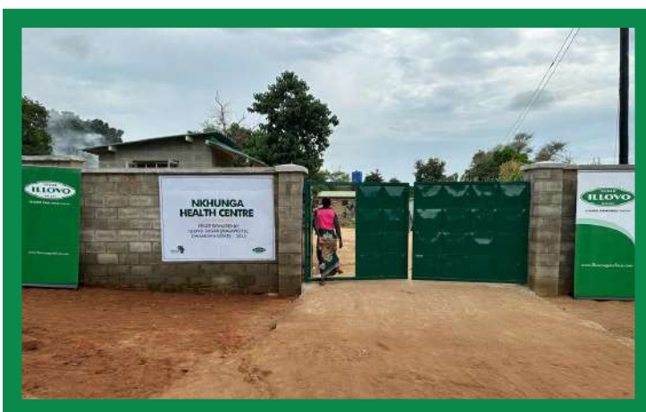
Entrance to Nkhunga Health Centre
